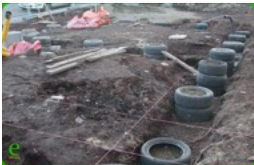
The above photograph depicts an Old Rubber Tire type of foundation under construction in the United Kingdom. Photograph sourced from: **inglepingle.co.uk**
