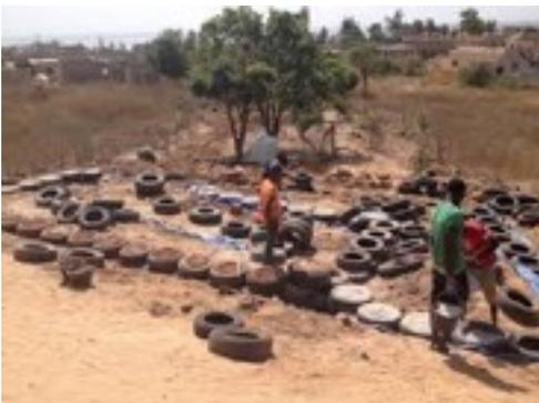
Photo at left depicts a gravel and old tire building foundation under construction. This photograph was sourced from: **abundantedge.com**
