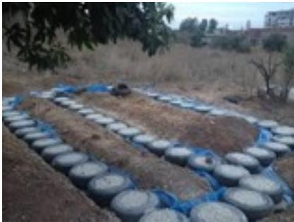
Photo at left shows a completed tire and gravel foundation ready for the next phase of building construction. This photograph was sourced from: **abundantedge.com**
